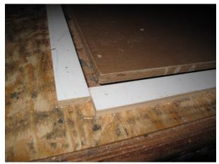
$\sim 3/32$ " as required, from all 4 edges of the hatch opening in the sole to make openings perfectly rectangular and clean. Had to remove NT installed hardware within the cut zone. Squared rounded corners left from the router bit radius by hand with chisels.
